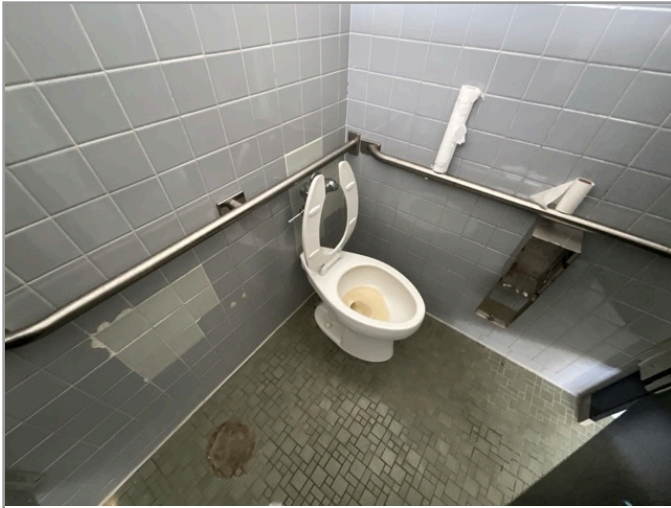
TOILET STALL OVERVIEW
