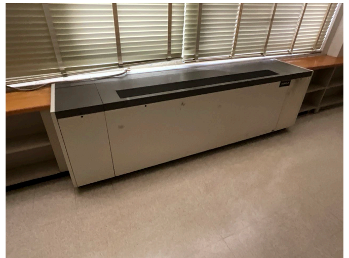
16 - TYPICAL UNIT VENTILATOR
