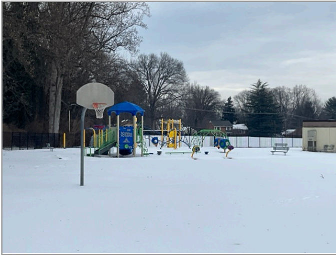
ACCESSIBLE ROUTE TO PLAYGROUND
