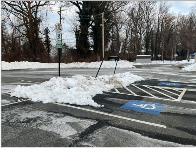
OVERVIEW OF ACCESSIBLE PARKING AREA
